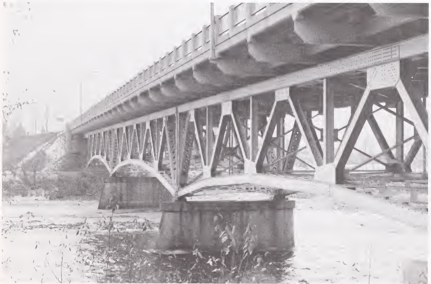
The Orange Street or Parkway Bridge in Missoula. The bridge is one of the more visible deck truss bridges in Montana.
